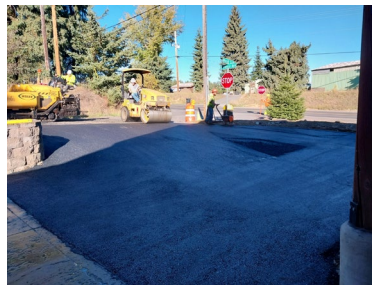
Paving the lower parking area at the Weippe Public Library.
