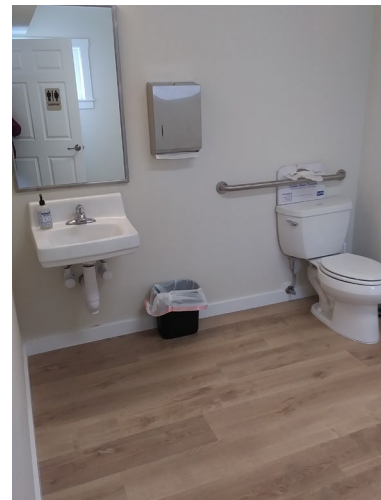
The new ADA-accessible restroom at the Wilder Public Library.
