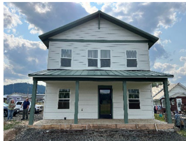
The exterior of the Benewah County Free Library District.
