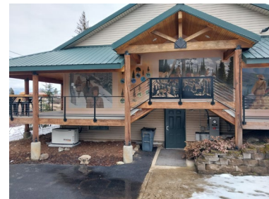
Completed paving, generator, one WiFi bar, and new railing at the Weippe Public Library.
