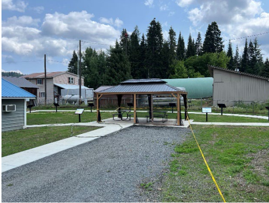
The new gazebo and covered seating area outside the Elk River Free Library District. The newly paved sidewalk connects the parking area, gazebo, and back library entrance.
