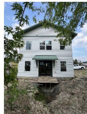
The exterior of the Benewah County Free Library District.
