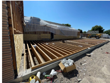
The Burley Public Library addition in progress.
