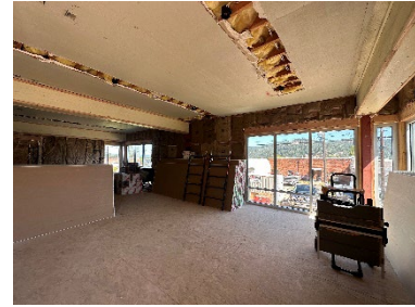
The interior of the St. Maries Public Library building during construction.
