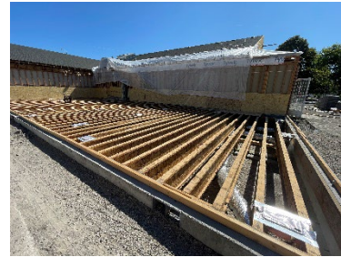
The Burley Public Library addition in progress.
