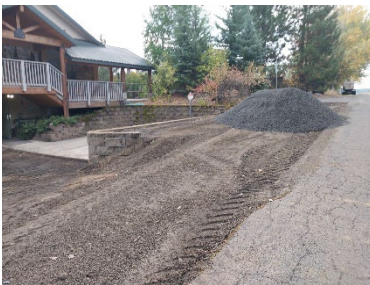
Preparing the area around the Weippe Public Library for asphalt application.
