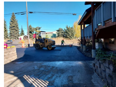
Paving the lower parking area at the Weippe Public Library.
